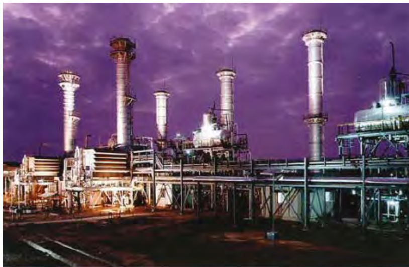
CHP Plant: Arvind Textile Mill, India
